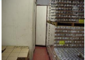
Obstructed Exit Route
